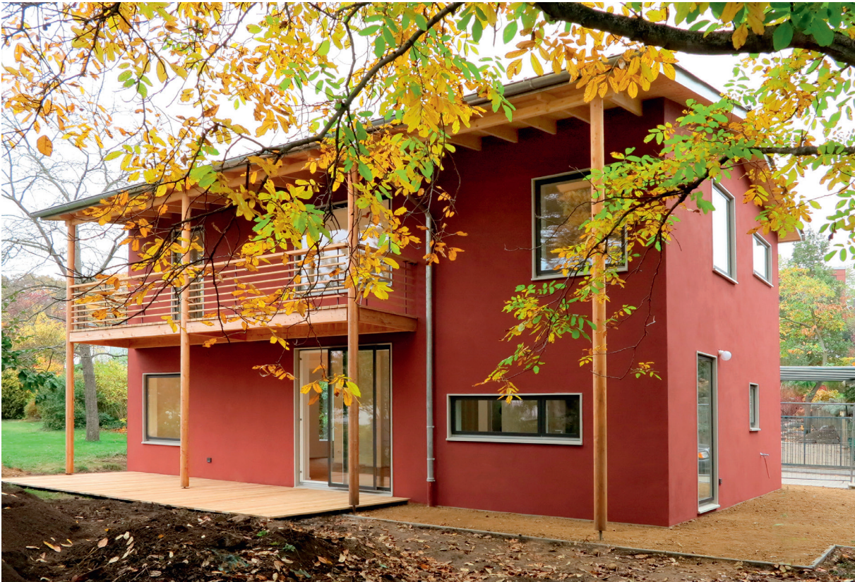
Figs. 3-6 Haus J, Darmstadt. 3: Completed building after a construction period of six months: the shell of heavy straw light earth is coated with a lime render. 4: The continuous earth shell enveloping the house took approximately four weeks to dry out. 5: Timber structure with a lattice of battens onto which the light earth is applied. The roof protected earth construction works from the weather. 6: Preparation of clay slurry from dry earth with a Knauf PFT G4 mixing machine.
