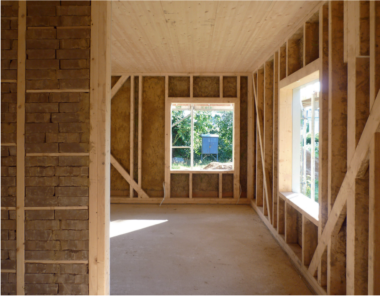
Fig. 8 Haus J, shell of construction seen from inside. Once dry, internal plasterboard is applied and the cavity filled with cellulose blow-in insulation. The internal walls are filled with dry-stacked earth bricks, i.e. without mortar.
