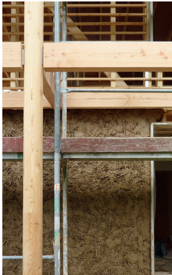
Figs. 3-6 Haus J, Darmstadt. 3: Completed building after a construction period of six months: the shell of heavy straw light earth is coated with a lime render. 4: The continuous earth shell enveloping the house took approximately four weeks to dry out. 5: Timber structure with a lattice of battens onto which the light earth is applied. The roof protected earth construction works from the weather. 6: Preparation of clay slurry from dry earth with a Knauf PFT G4 mixing machine.
