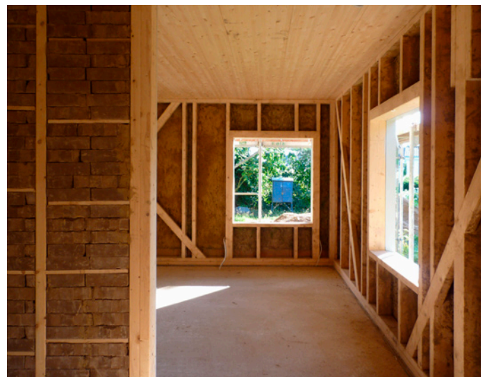
(10) In the renovation of half-timbered houses, the homogeneous brick lining with light earth blocks is the state of the art.
