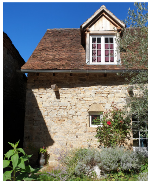
(4) Repair of straw-clay fillings. Intact parts are preserved and the missing parts are completed with reclaimed material (5) Stone masonry with earth mortar in the Dordogne.
