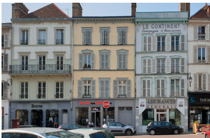
(6) Plastered wood+earth buildings in the city centre of Troyes
